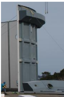
Figure 3-4. Detail from picture of Aquafarm CCS under construction possibly showing integrated GRP buoyancy ring
