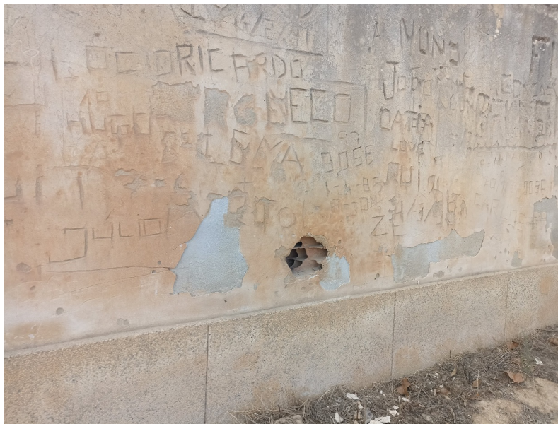
Figure 2. Detail of the wall with bricks and mortar
