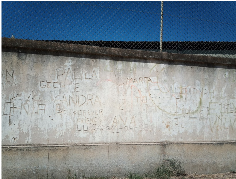
Figure 4. Engravings on the wall with personal names
