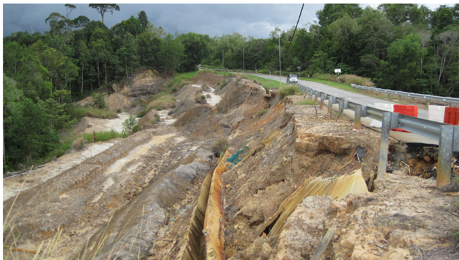
Fig. 2 An illustration of the severity of erosion process, if soil is not protected from rainfall. Labi Road, Brunei Darussalam. Photo: K. Becak
