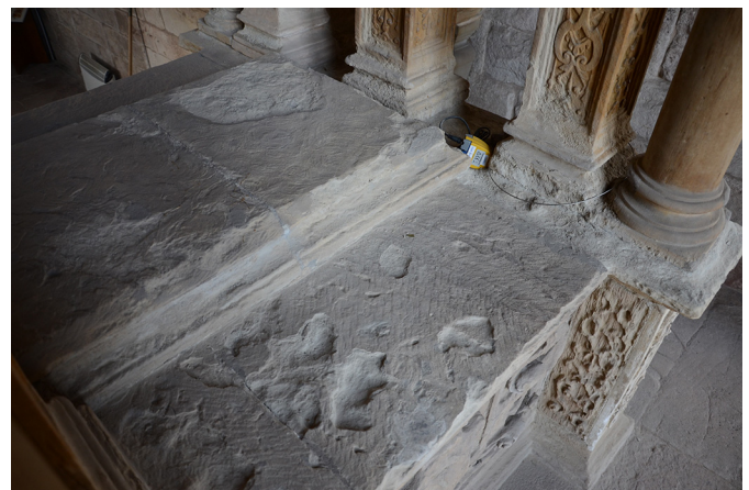
Fig. 5. Decay on the top of the tomb at the Skelmorlie Aisle, Largs. Here the dense fine-grained sandstone is suffering from cratering and powdering. At the centre top right of the image, an environmental logging device can be seen attached to the structure, recording conditions of Temperature and Relative Humidity near to where the damage is occurring (Photograph: Maureen Young, Historic Environment Scotland).
