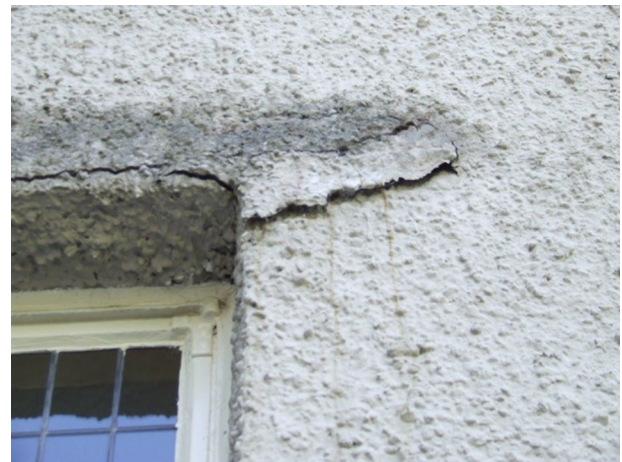
Fig. 7. Example of the cracking in the Portland Cement render of the Hill House, Helensburgh. Cracking such as this allows water ingress that threatens the historic Macintosh-Macdonald designed interior decoration and furniture (Photograph: John Hughes).
