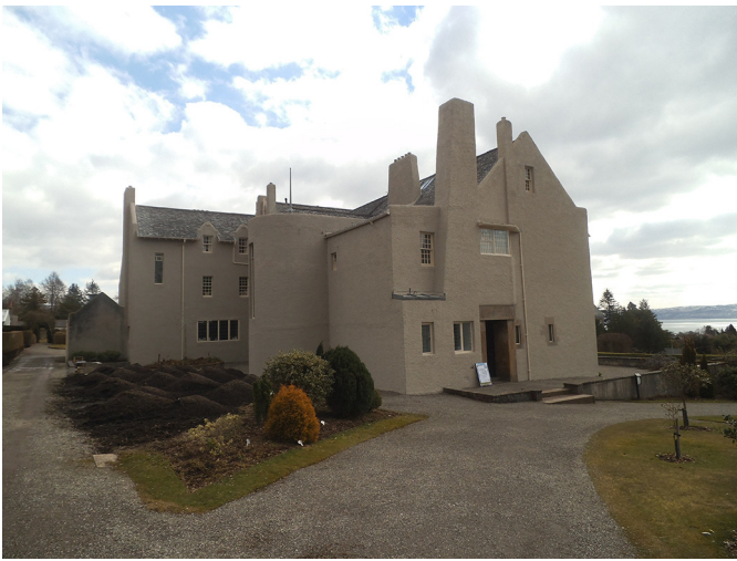
Fig. 6. The west façade and the entrance to the Hill House, Helensburgh, Argyll and Bute (C.R. Mackintosh, architect, 1904–5). This view was taken in 2013 some months after the exterior Portland Cement render had been painted to unify the appearance and improve resistance to environmental attack. The Clyde estuary can be seen in the background (Photograph: John Hughes).
