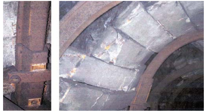
Figure 5. The displacement in the yielding steel sets and deformation in struts on the beneath level of the fractural zone (level 2200 m).
