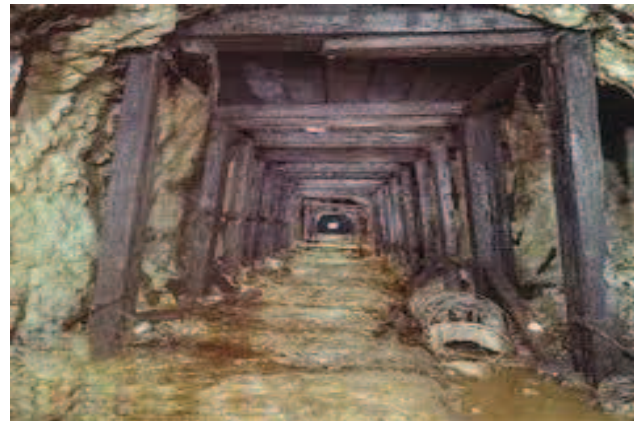
Figure 3. Timbering in tunnels.
