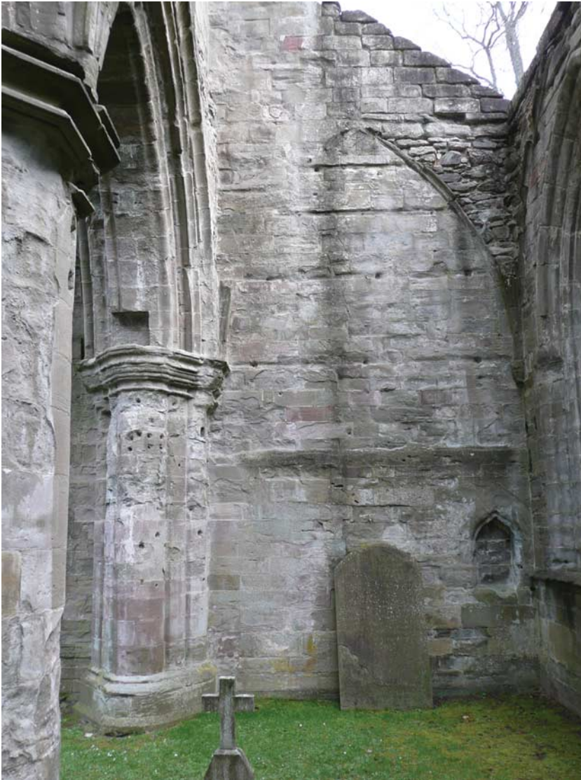
Fig 30. Dunkeld cathedral: east wall of the south nave aisle. The horizontal chases in the wall are perhaps for the fixings of an altar retable; a piscina is seen to the right
