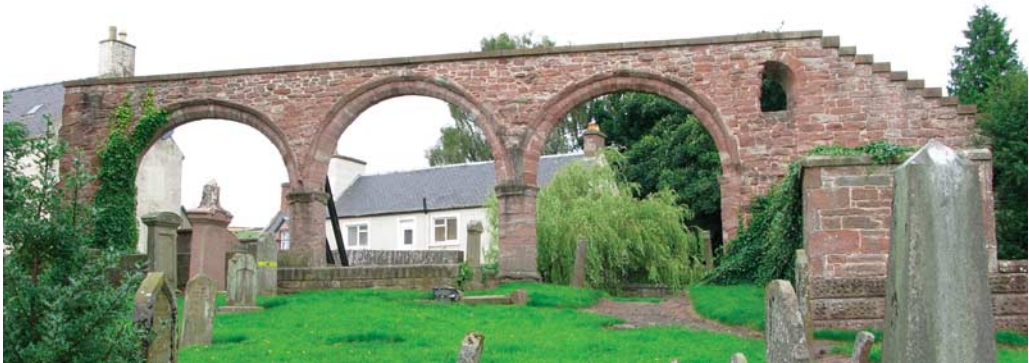
Fig 20. Alyth church: the surviving late medieval north arcade from the south. This was preserved after a new church was built in 1836 because it was believed to be 'in the Saxon style of architecture'
