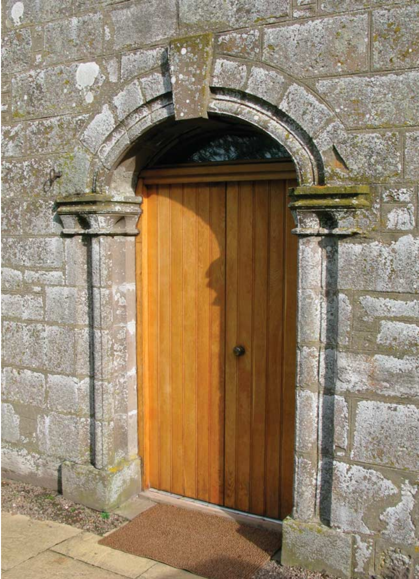
Fig 29. Auchterhouse church: south nave doorway. This appears to incorporate late medieval jamb and arch mouldings within a doorway of 1775
